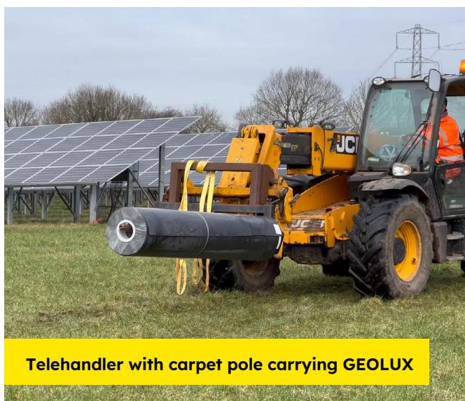
A properly structured and supported pole can be used to unload **GEOLUX** rolls onsite. As an alternative, straps that are appropriately rated can be used as a Solmax approved lifting method to unload **GEOLUX** rolls. Lifting straps are supplied on every roll. Each **GEOLUX** roll label contains roll weight information that should be consulted in determining appropriate lifting equipment and factors of safety.
