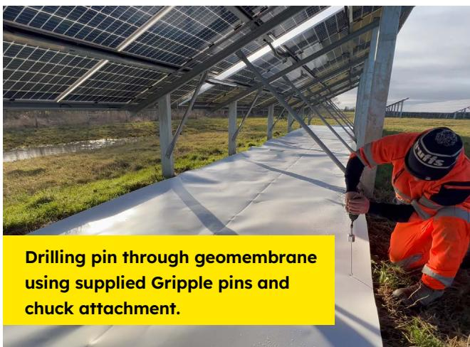
**Drilling pin through geomembrane using supplied Gripple pins and chuck attachment.**
