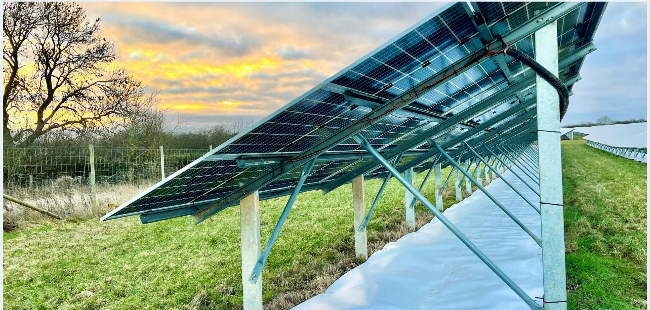
**GEOLUX®** provides a maximized level of Solar Energy Reflectance to increase the ground albedo to approximately 75%, resulting in an optimum increase in the power gained from bifacial solar panels.
